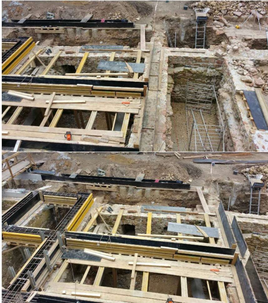
Fig. 13. Construction of the floor slab over the uncovered medieval cellars under the courtyard (Photo by the author)
