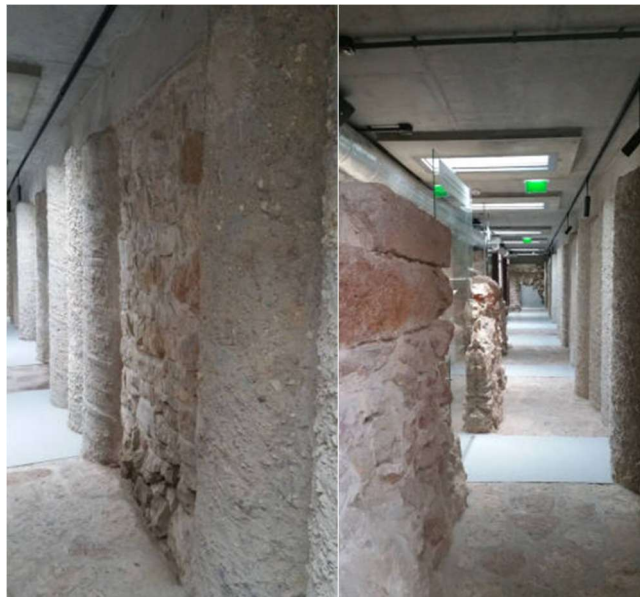
Fig. 19. Cellars under the courtyard, after uncovering and renovation. Palisade retaining wall – detail (on the left). The permanent exhibition rooms, naturally lit by skylights (on the right) (Photo by the author)
