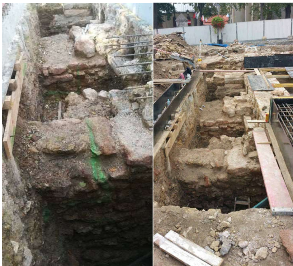
Fig. 12. Construction of load-bearing beams for the courtyard slab (at the same time - the floor slab above the medieval cellars) (Photo by the author)
