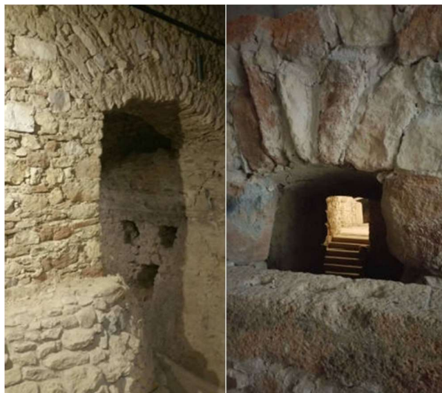
Fig. 17. Cellars after uncovering and renovation (Photo by the author)
