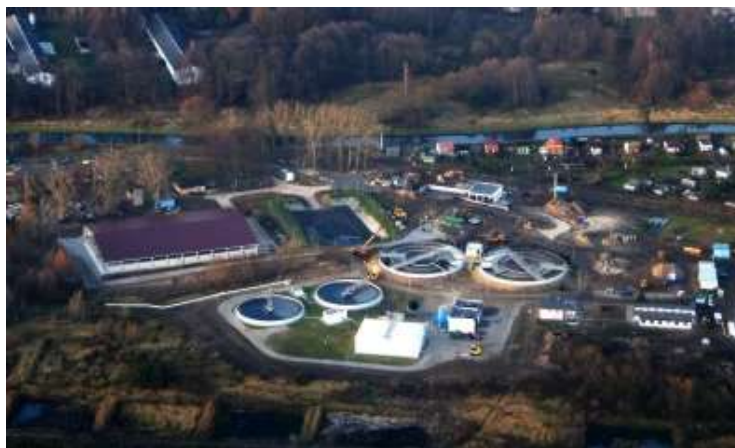
Fig. 1. Wastewater treatment plant in Goleniów
