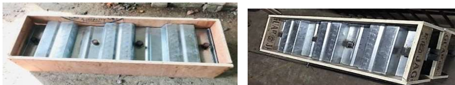
Fig. 2. Formwork for the specimen with welded decking sheet and shear connectors
