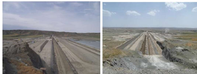
Fig. 2. Construction of the Sumbar Dam
