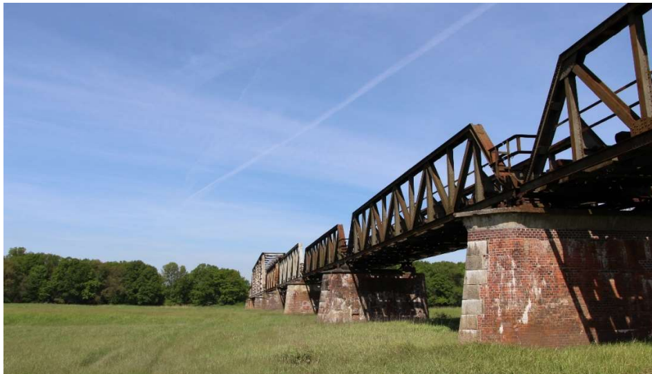
Fig. 3. View of the bridge from the eastern side (photo by the Author, 2017)
