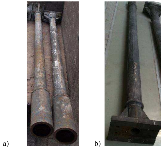
Fig. 4. The cast iron columns before a) and after b) reinforcement
