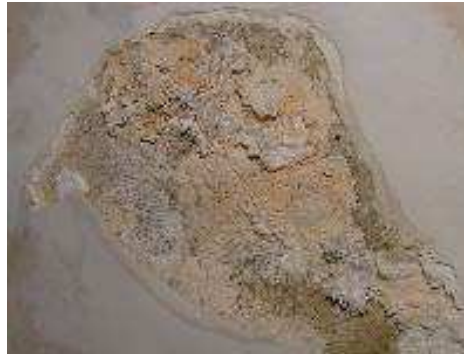
Fig. 2. Crystallization of the salt within the plaster
