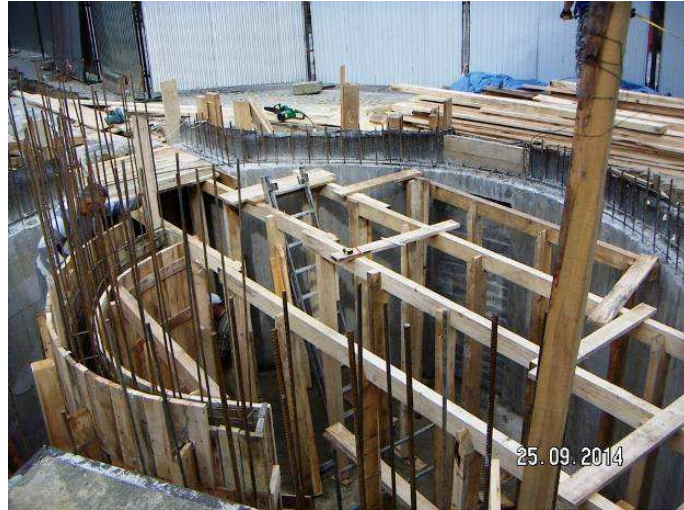
Fig. 5. Przemyśl – implementation of the underground rotunda - the entrance to the underground tourist route (photo by UM Przemyśl)
