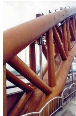
Fig. 29. Truss concrete filled steel tubular (CFST) through bridge of 200 m span, near Quilin (China)
