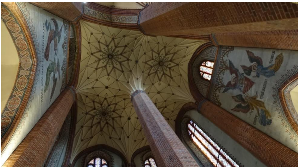
Fig. 11. Diamond vault over a northern part of the transept in Cistercian Abbey in Pelplin
