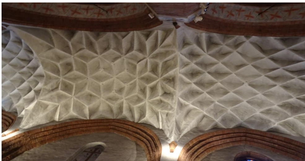
Fig. 14. Diamond vaults over an aisle in St. Jacob's Basilica in Olsztyn
