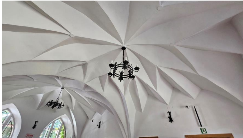
Fig. 17. Diamond vault in the buildings of the former Dominican monastery in Myślubórz
