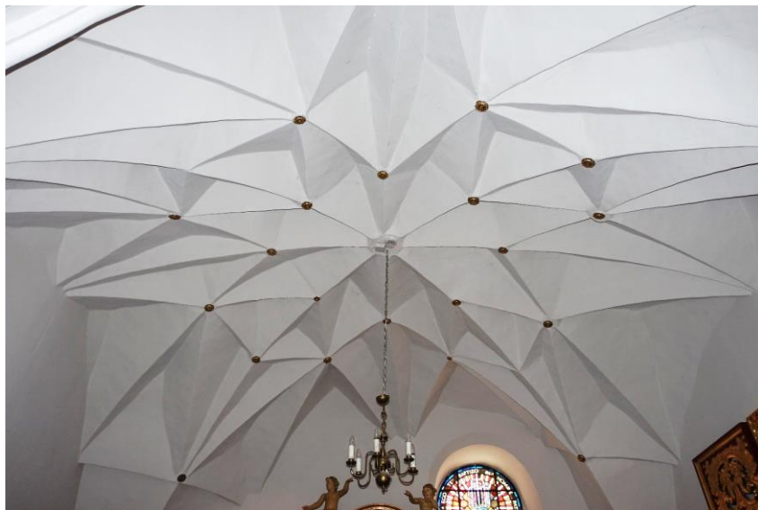
Fig. 18. Diamond vault in the church of St. Michael the Archangel in Świebodzin
