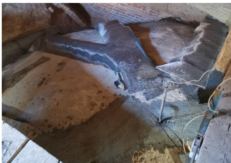
Fig. 29. Application of the FRCM system to top ribs in the rib vaults in St. John's Church in Malbork (photo by M. Jackiewicz)
