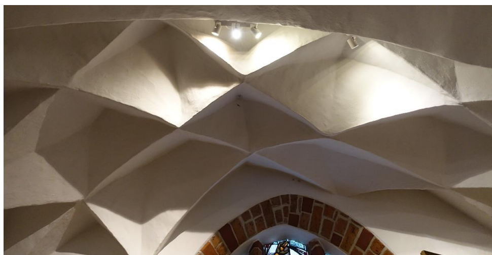
Fig. 16. Diamond vault of one of the chapels of the church of St. John the Baptist in Stargard
