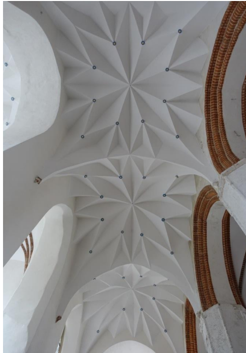
Fig. 7. Diamond vaults over an aisle in St. Catherine's Church in Gdańsk
