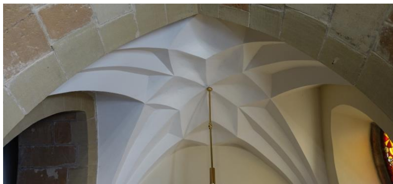
Fig. 21. Diamond vault in part of the porch in St. Margaret's Basilica in Nowy Sącz
