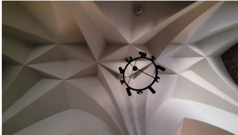
Fig. 19. Diamond vault over the porch in the Cathedral of Holy Cross in Opole
