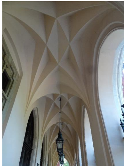
Fig. 20. Diamond vaults in Cracow: a) Collegium Maius, b) Collegium Novum
