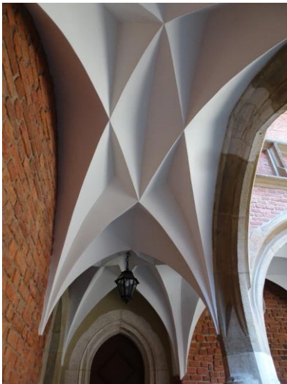
Fig. 20. Diamond vaults in Cracow: a) Collegium Maius, b) Collegium Novum
