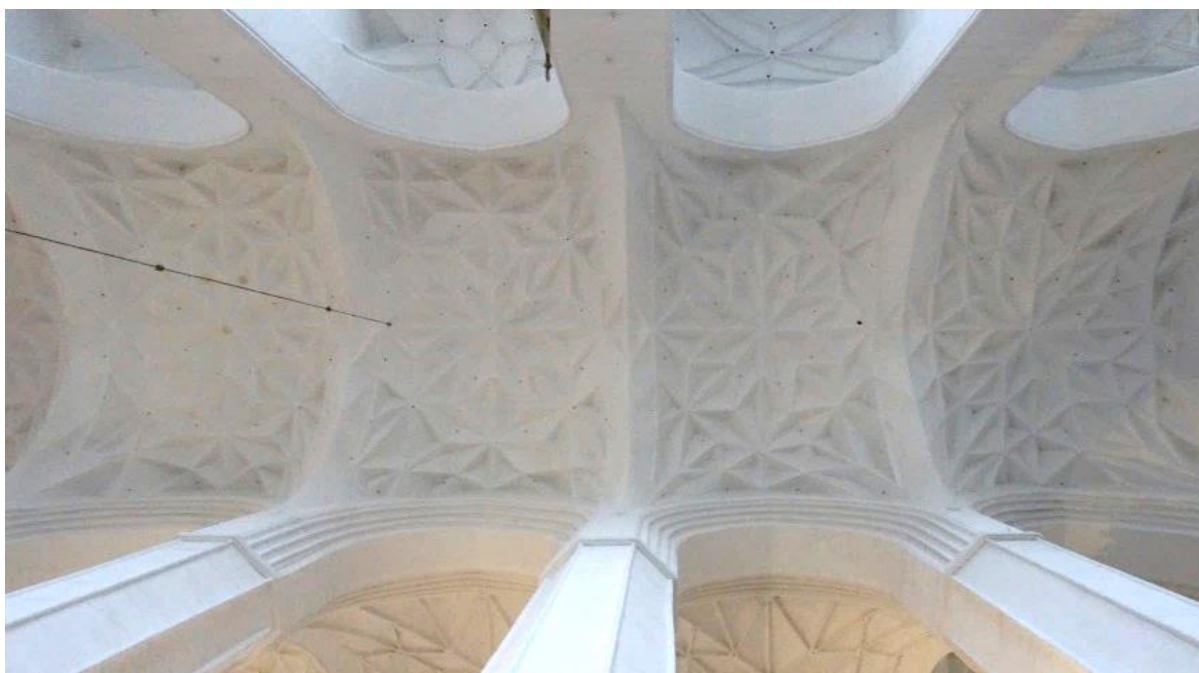
Fig. 6. Diamond vaults over aisles in St. Mary's Basilica in Gdańsk
