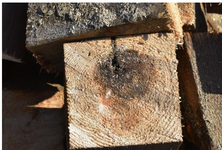
Photo 7. Internal damage to the wooden element
