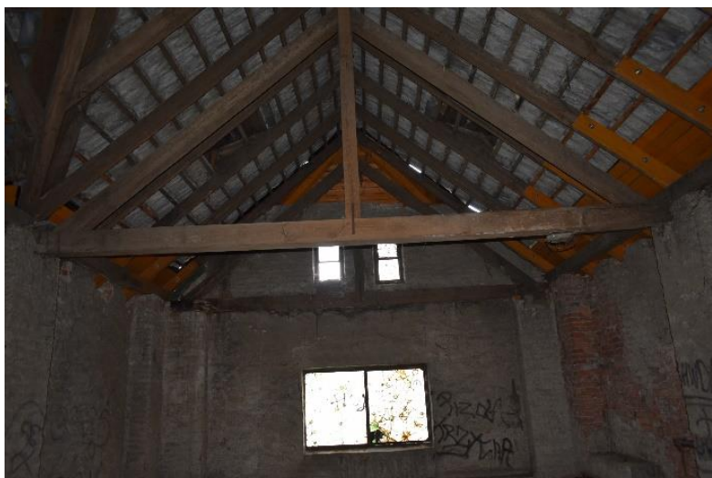
Photo 6. Roof truss in segment D
