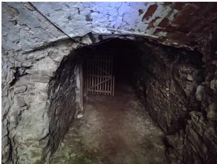
Photo 4. Vaulted basement of the Kossak Manor Granary building
