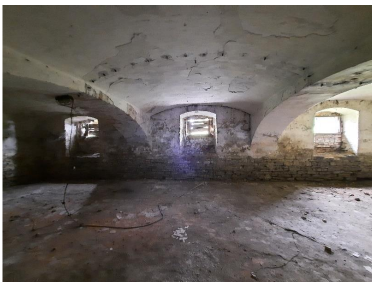
Photo 5. Basement with barrel vaults supported by transverse arches
