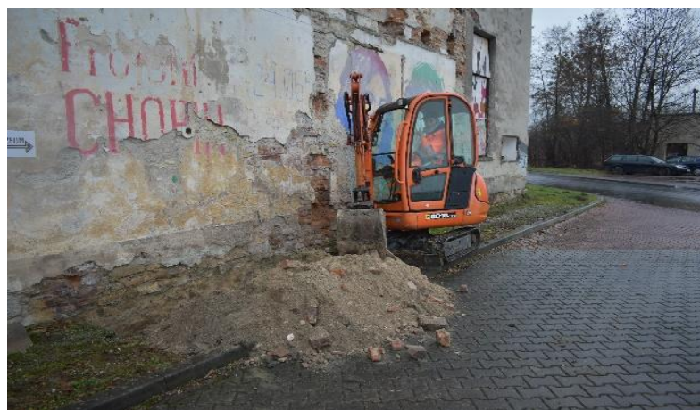
Photo 11. Damage to external walls
