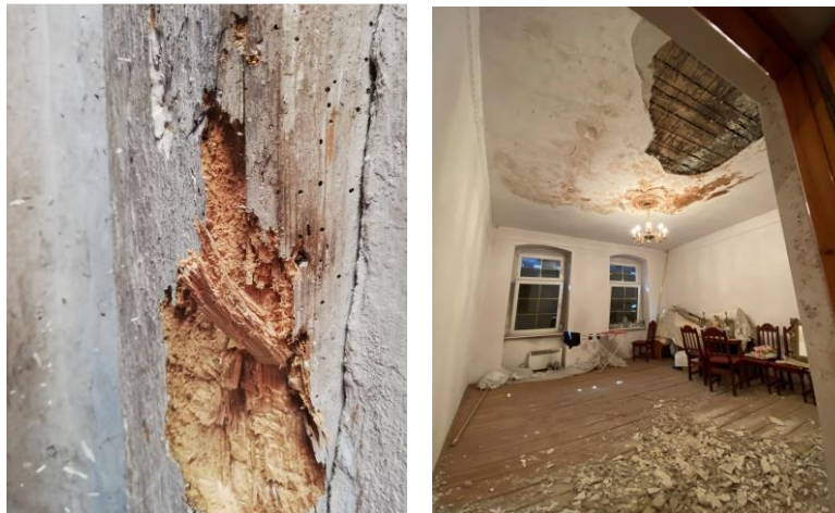
Fig. 4. View of contaminated surfaces after application of the natural drainage method
