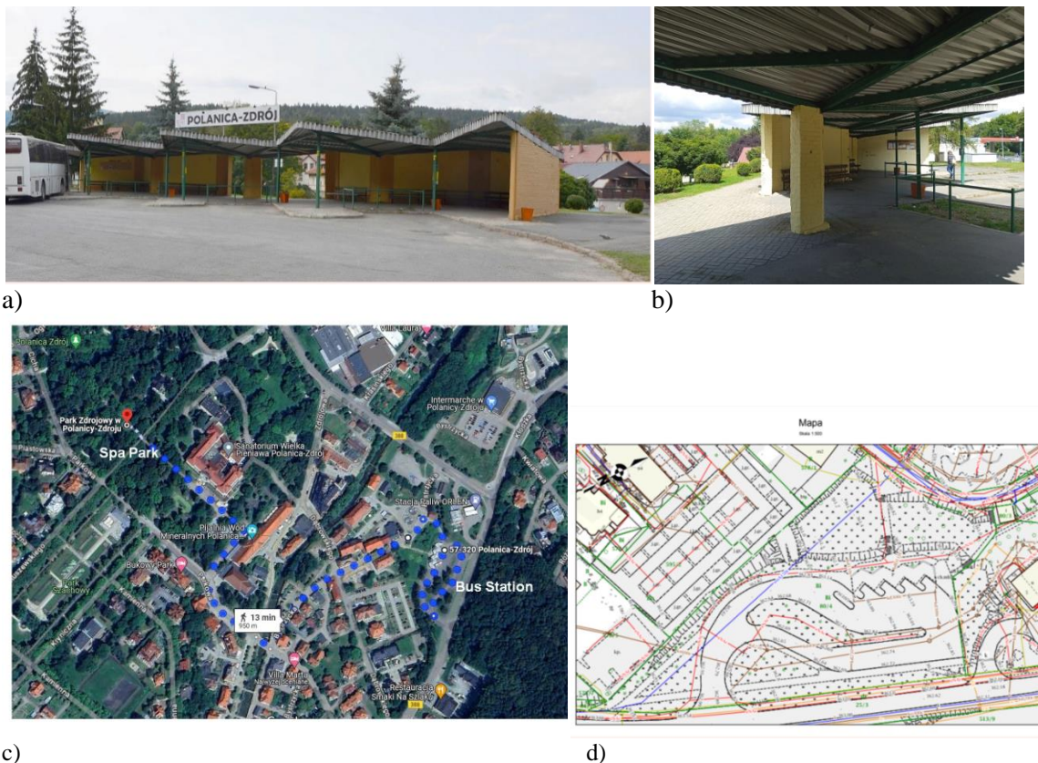
Fig. 2. Bus station in Polanica-Zdrój a),b) Technical condition of the bus station in Polanica-Zdrój, (2023) c) station area on the side of the pedestrian zone of the city centre, Spa Park, (700-900m on foot),source: google map d) bus station plan
