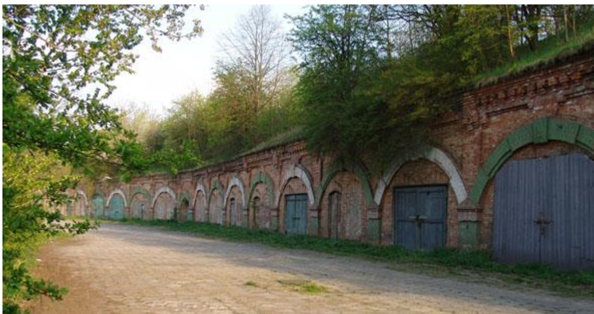
Fig. 4. Condition before the revitalisation of Fort Służew. Source Festgrupa
