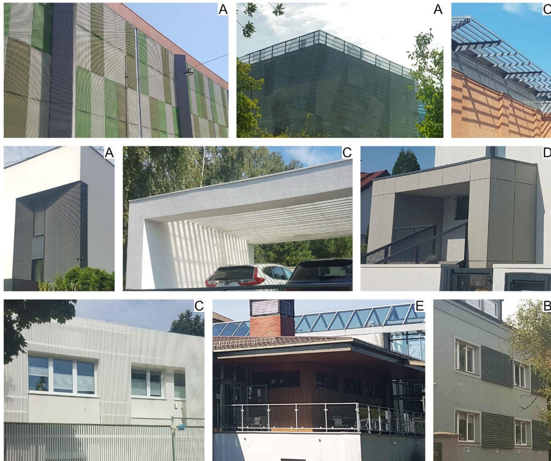
Fig. 1. Examples of covers shading an opaque facade: A – openwork sheets, B – blinds, C – boards, strips, D – boards, E – eaves (photo by M. Siewczyńska)
