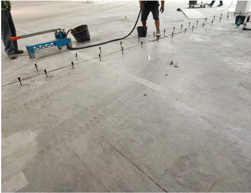
Fig. 16. Concrete industrial floor (Example 4) during repair: installation of packers and feeding of cement injection with a pump [38]
