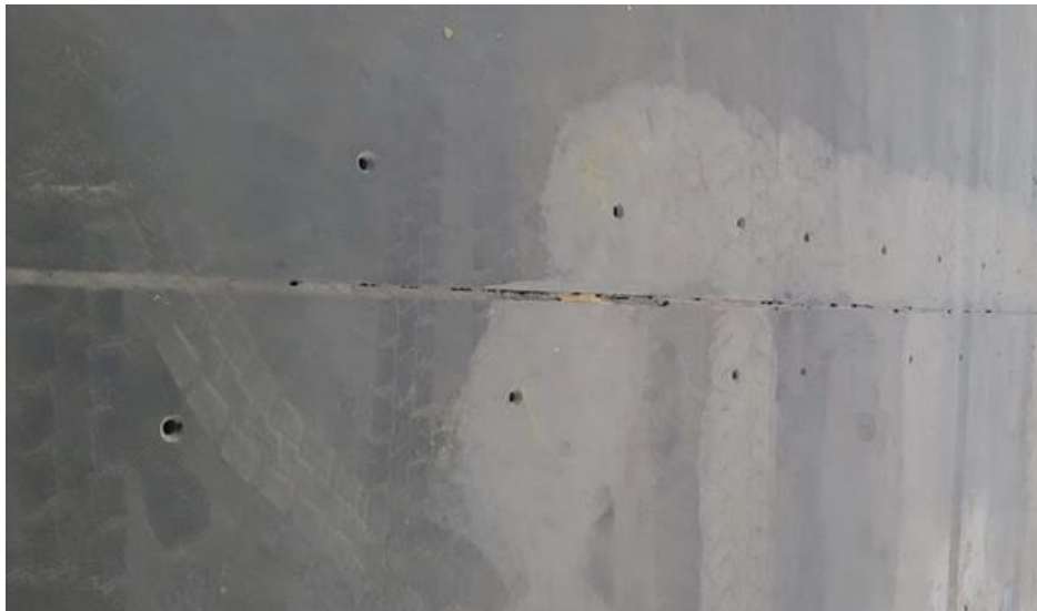
Fig.15. Concrete industrial floor (Example 4) during repair: diagram of drilled holes for injection feeding [38]
