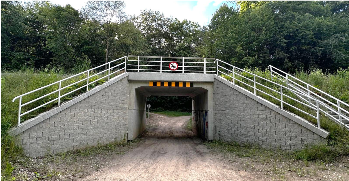
Fig. 4. A view of the bridge from the south-east after renovation
