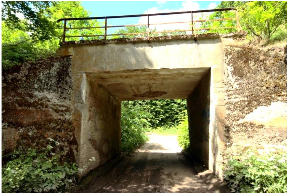
Fig. 1. A view of the bridge from the south-east
