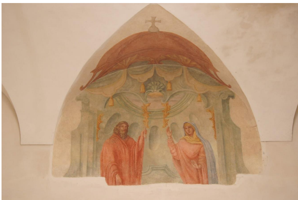
Fig. 25. Entrance to the former chapel after the completion of conservation works, photo by K. Janus, 2023
