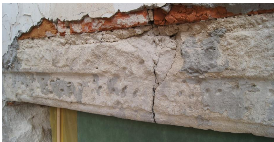
Fig. 8. Remains of the preserved stone lintel of the window surround in the courtyard, photo by K. Janus, 2024
