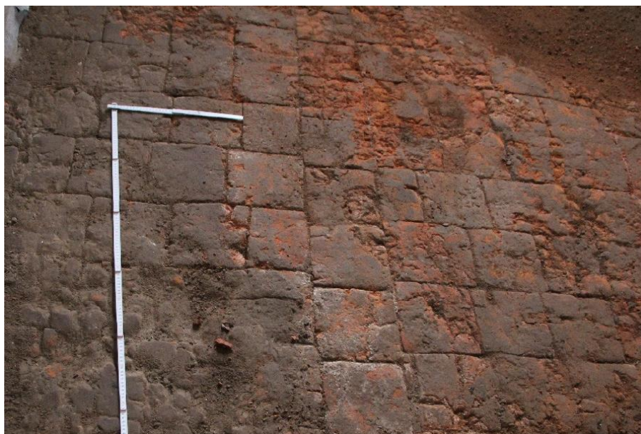
Fig. 14. Fragment of a brick floor from the 17th century in the corridor, photo by K. Janus, 2023
