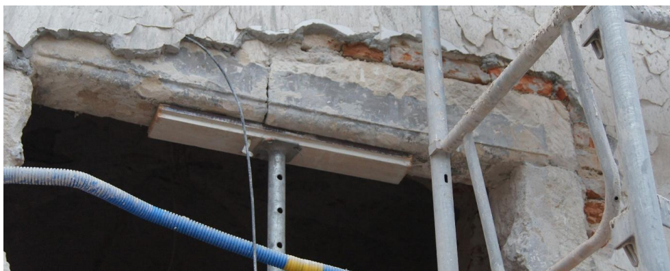
Fig. 9. Remains of the preserved stone lintel of the window surround in the courtyard, photo by K. Janus, 2024
