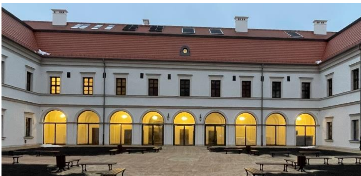
Fig. 7. View of the academy courtyard from the east after the renovation works were completed, photo by K. Janus, 2024
