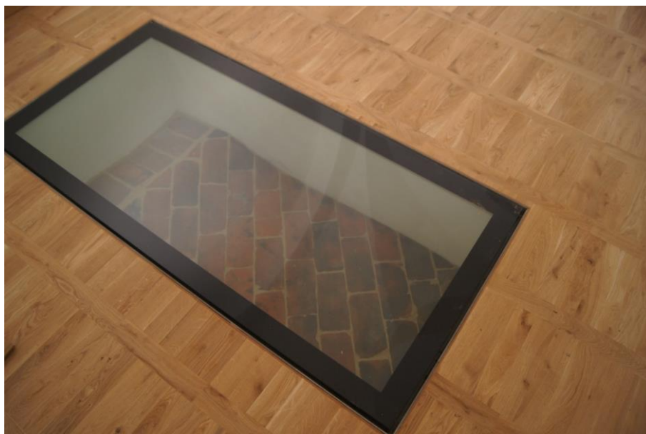
Fig. 13. Floor of a residential/craft building from the 16th century after cleaning and exhibition, photo by K. Janus, 2023
