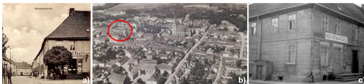
Fig. 2. Corner of the building facing the market square on a postcard from 1913.: a), Location of the building within the urban fabric of Myślubórz (highlighted in red) in 1945.: b), Condition of the building in an archival photograph from the 1960s. Source: postcard (a) and photograph (b - c) from the authors' archives
